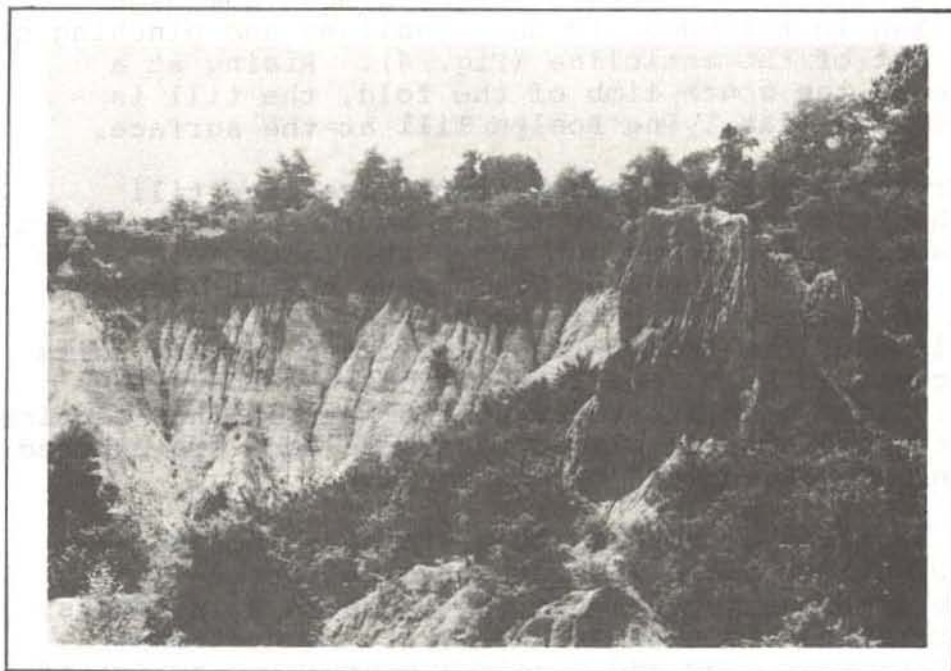
Figure 3D. P.W., Stop 2B - Large, eroded pinnacle of resistant Montauk (?) Till at right is partially covered by ice-shoved Cretaceous sediments seen as light area in cliff (center & left). Horizontal Roslyn Till (5m) caps the section.
