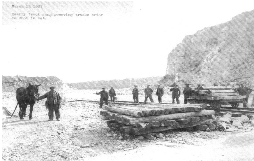
Figure 4. Moving railroad track at Universal Atlas Greenport Quarry in 1937.
