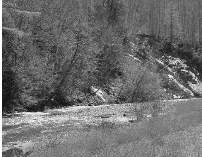
Figure 18. Pre-restoration landsliding along right bank of Stony Clove at Lanesville site. Photo from DuBois, 2003.
