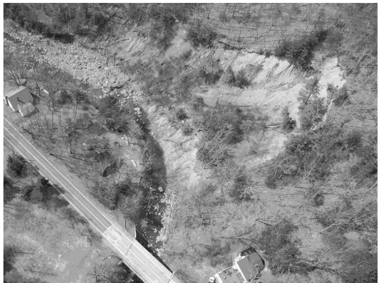
Figure 22. Landslide along Beaver Kill. Stop BK2 at bridge. Photo from NYCDEP et al., 2007.
