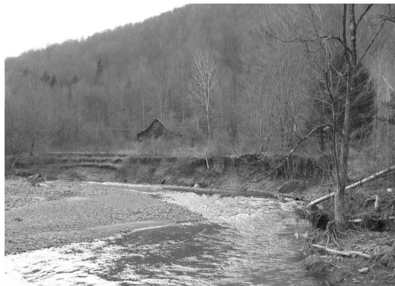
Figure 15. View upstream toward actively retreating streambank with rotational failure scarps exposed in adjacent terrace (photo courtesy DEP, 2006).
