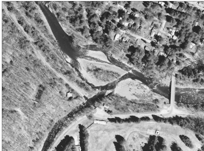
Figure 10. Aerial photo of the Woodland Creek/Esopus Creek confluence. The project reach extends from the head of the bifurcated reach down to the Woodland bridge (2001, DOQQ)
