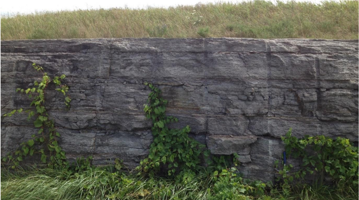
Figure 13. Southwest face of a road cut showing planar bedding in dark gray quartz arenite in the lower Theresa Formation. Stop 6, Chippewa Bay, New York.
