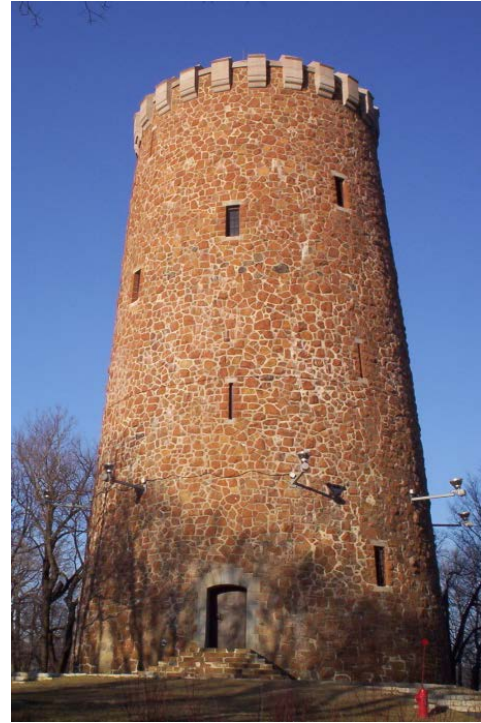
Figure 21. Tour Lévis, which occupies the summit of the higher hill, was constructed using the diatreme breccia.
