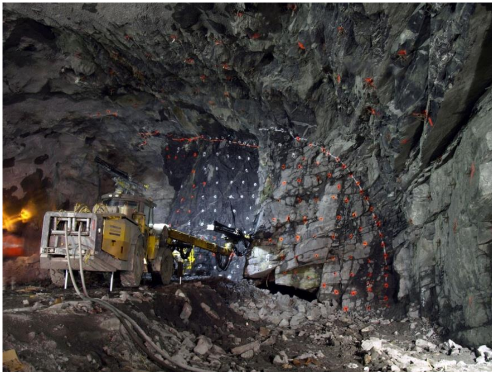
Figure 12 - View from north of west (R) and center (L) slashes of North Cavern excavation at 86 th Street Station for Second Avenue Subway. West (southbound) TBM tunnel crown at +77.2' exposed in right center of image below area of intersecting joints, faults and resulting overbreak. The center (wet, blackish area) and western (right of center) slashes are discussed in text. (Digital image taken 19 December 2012.)
