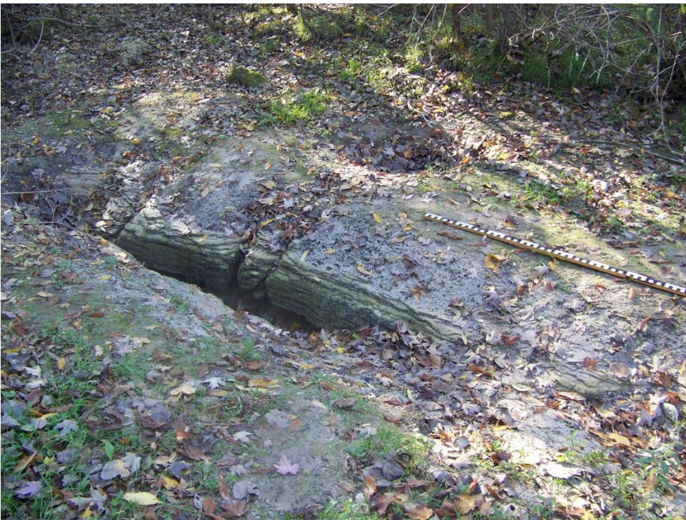
Figure 11. Photo of one of the many large open fractures that underly Mackay Spring.
