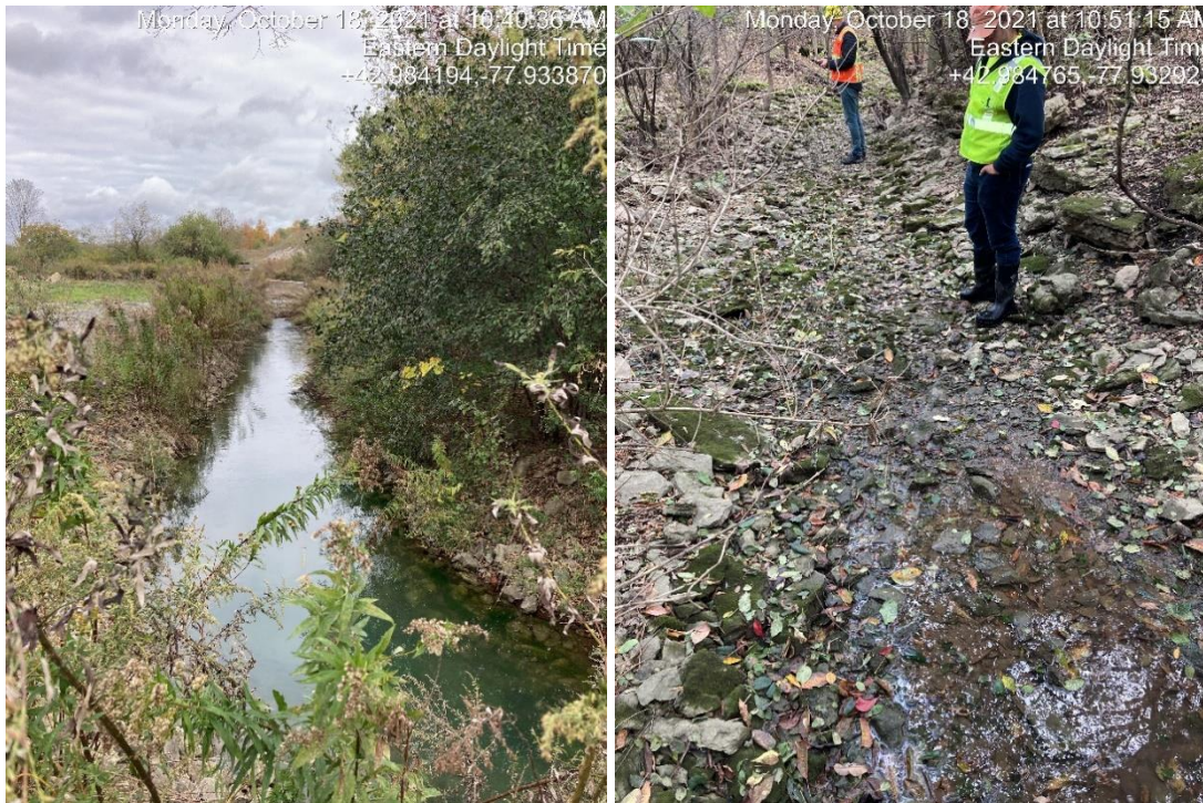
Figure 6. Dolomite Products SPDES outfall into Mud Creek (left). Discharge disappearing into the Mud Creek streambed a few hundred meters downstream of the outfall (Right).
